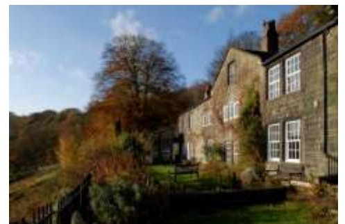
Lumb Bank, The Ted Hughes Arvon Centre, Yorkshire
